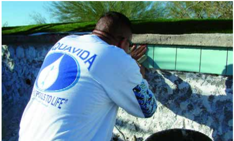
As good fortune would have it, we were able to find an exact replacement for the original waterline tile and, on our second day on the job, meticulously set the new tiles in place. We did all we had to do to make our work befit the pool – a key visual component of a national architectural treasure.
